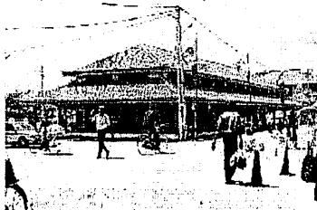
Newly renovated food market, built in the Dutch period (Prasad Amarasooriya, 1998)
