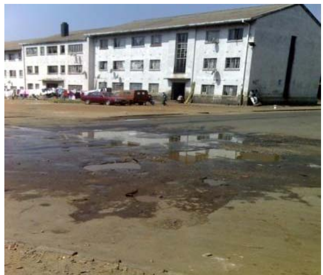
Fig 3: POTHoles FILLED WITH RAINWATER
