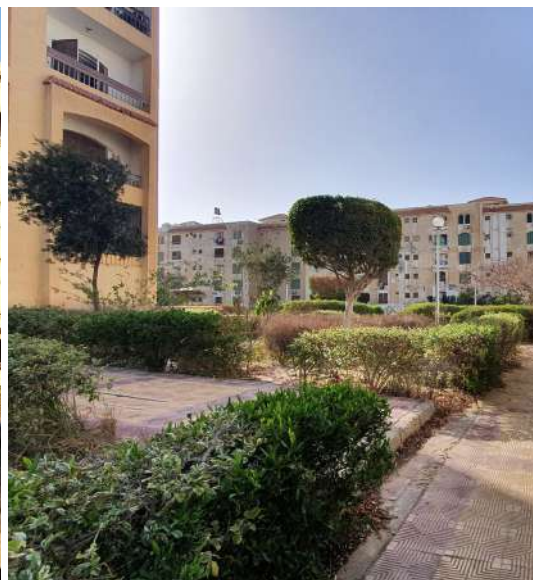
Figure 5.5: Zone A, Tatweer Housing in New Cairo.
