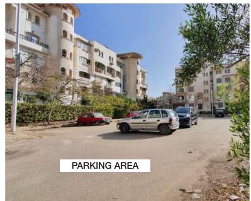
Figure 5.16: Zone A Tatweer Housing parking areas
