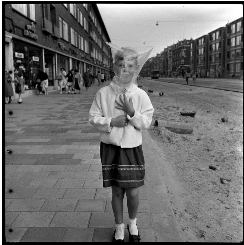
(Fig .03 - Netty van Aalst During Roadworks on Schiedamseweg. Netty van Aalst stands with a plastic bag over her head to protect herself from blowing sand during roadworks, 1956 - Source: Stadsarchief Rotterdam 2025)
